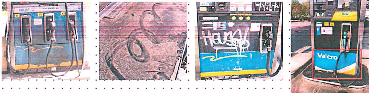
NOZZLES DAMAGED, OR EXCESSIVELY DIRTY
